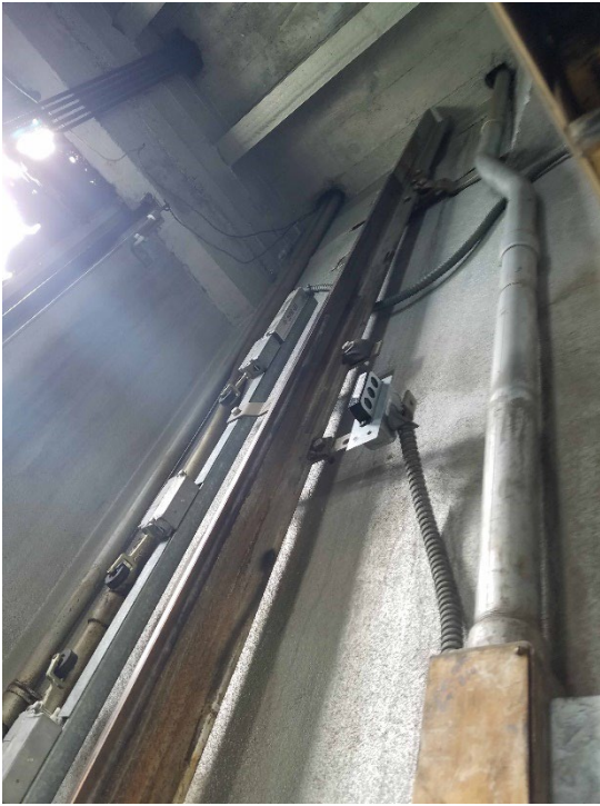
Photo 5: Existing elevator rail.
