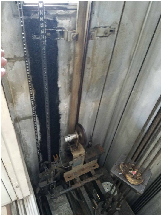
Photo 3: Existing elevator rail.
