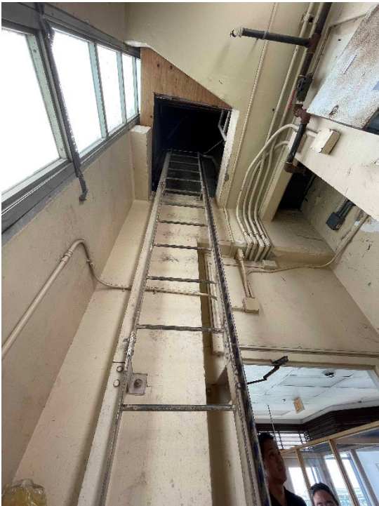
Photo 15: Ladder to elevator equipment room.
