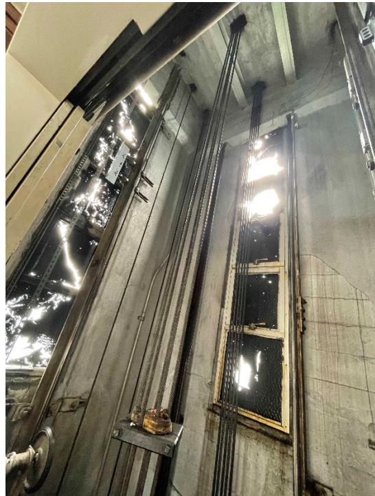
Photo 8: Existing hoistway.
