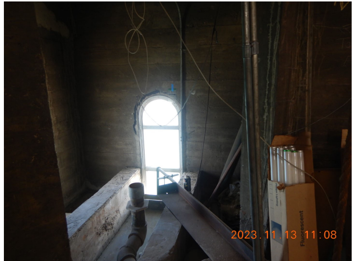
Photo 21 - AT-11-M-03C (Panoramic) [AL\DSCN2091.JPG]
