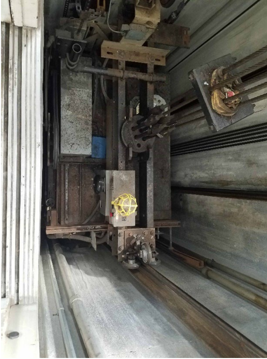
Photo 1: Top of existing elevator cab.
