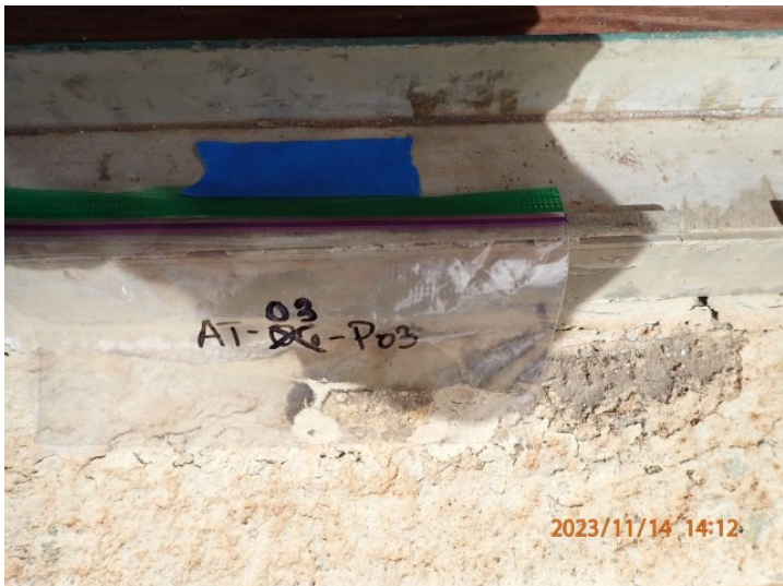
Photo 40 - AT-03-P03 (Close-Up) [JV\JVAL1608.JPG]
