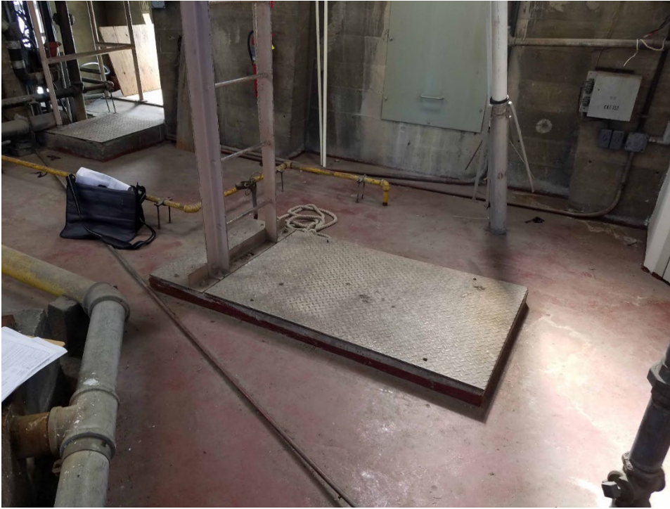
Photo 23: Diamond plate cover over access hole to floor below.
