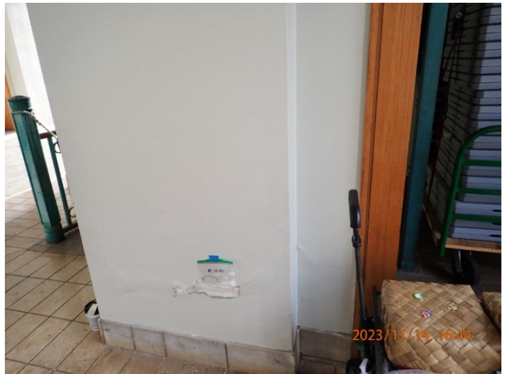
Photo 23 - AT-GF-P01 (Panoramic) [JV\JVAL1646.JPG]
