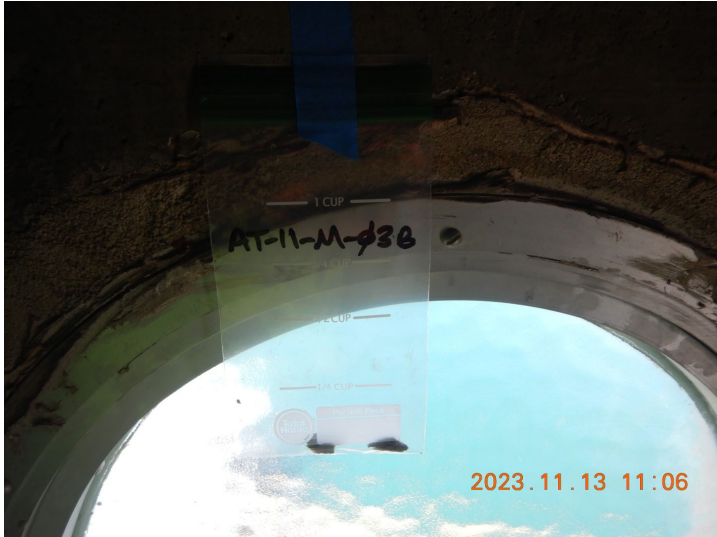
Photo 18 - AT-11-M-03B (Close-Up) [AL\DSCN2088.JPG]
