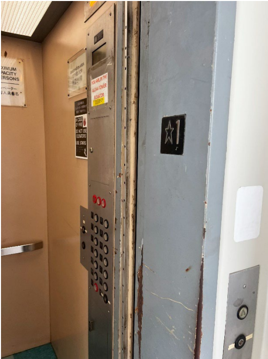
Photo 13: Existing cab jamb.
